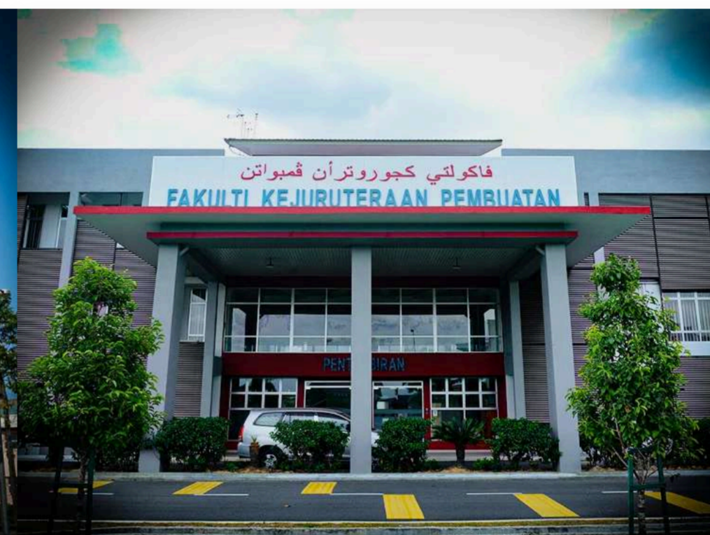
Faculty of Industrial and Manufacturing Technology and Engineering (FTKIP)
